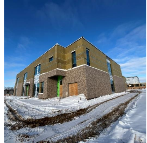
Construction progress on the new north Regina joint-use school.
