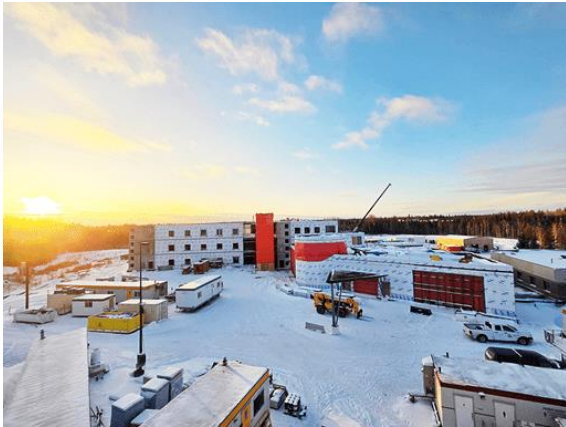
Construction progress on the La Ronge Long-Term Care home.
