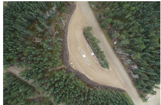
Drone footage of the new trailer sewage dump which will be located at Narrow Hills Provincial Park.
