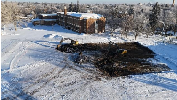
Site work for the Saskatoon Urgent Care Centre.
