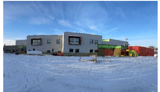
Construction progress on the new CÉF Regina school.
