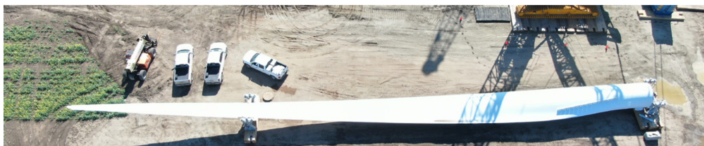
GOLDEN SOUTH WIND ENERGY FACILITY CONSTRUCTION
