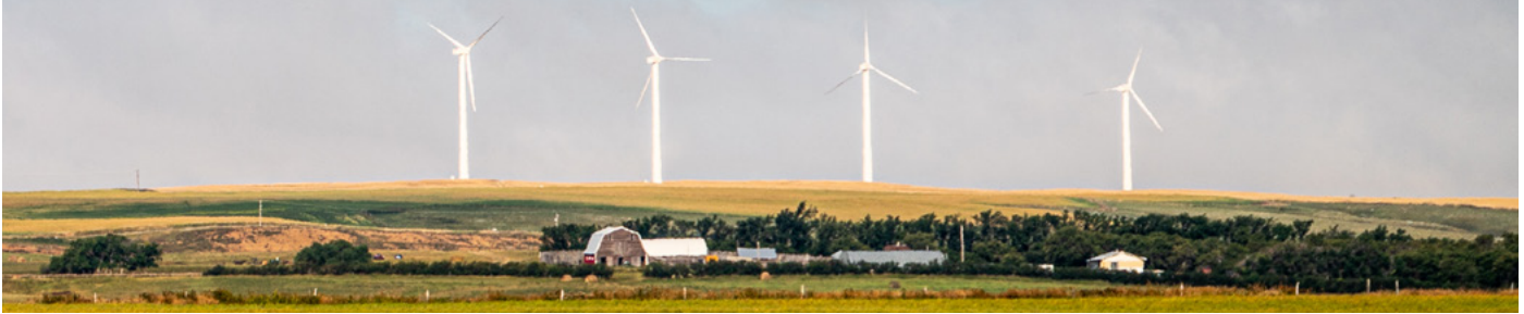
CYPRESS WIND POWER FACILITY
