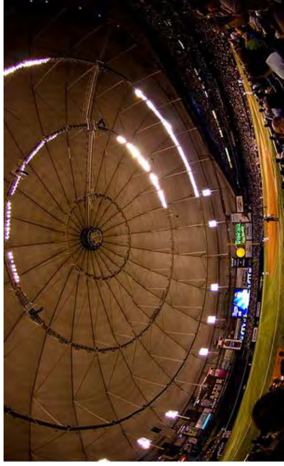
Tropicana Field, FL (45,369) Tension/ Compression Ring
